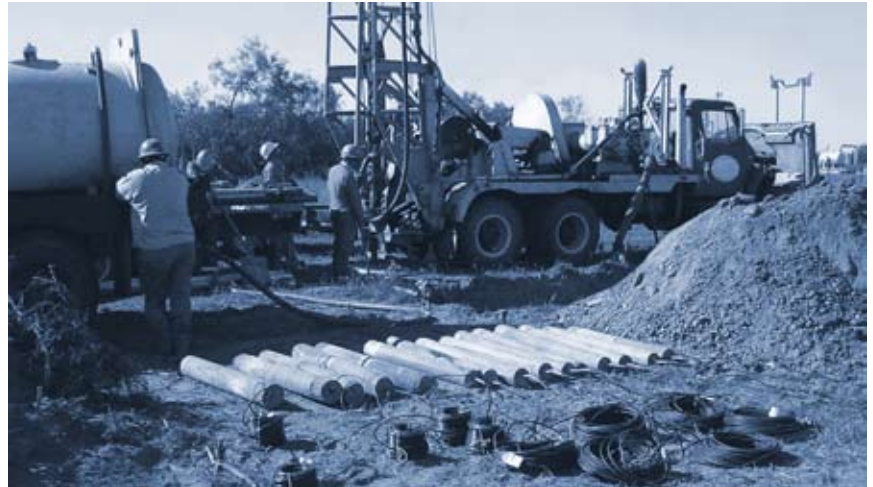
EnvirAnode® installation using familiar drilling, mixing and pumping tools and techniques
