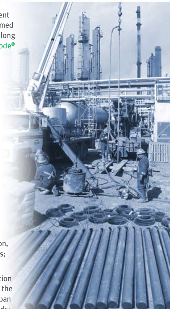
EnvirAnode® installation at an oil refinery
