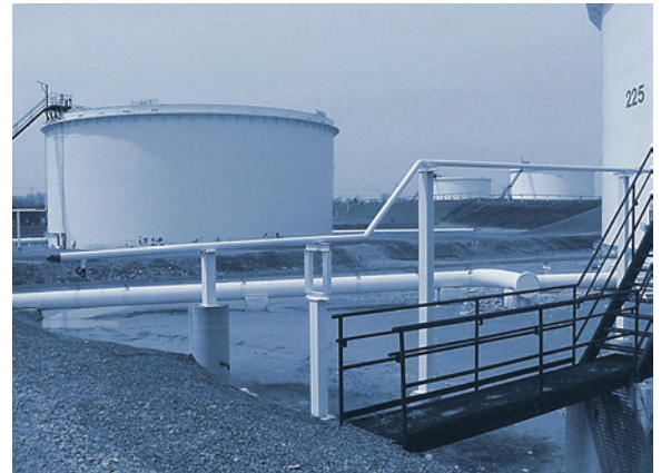
Closer view of storage tanks and associated infrastructure
