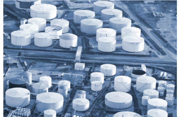
Dense tank farms present major grounding challenges
