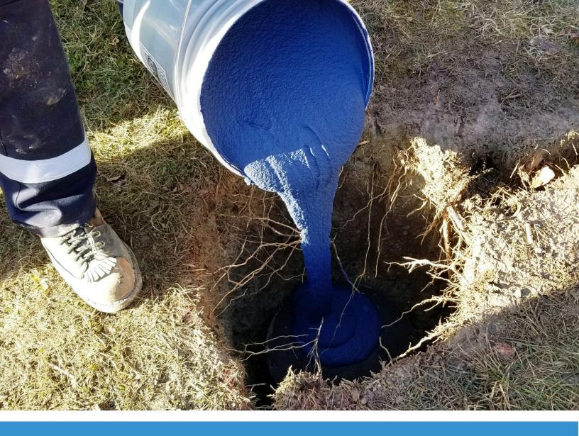
**ConduFlow®:** A low dust approach to electrical and utility grounding
