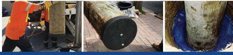
The **ConduDisc**<sup>®</sup> can be used with or without **ConduFlow**<sup>®</sup> pourable backfill. When using **ConduFlow**<sup>®</sup> with the **ConduDisc**<sup>®</sup>, ensure that **ConduFlow**<sup>®</sup> is properly mixed and poured down the hole prior to installing the **ConduDisc**<sup>®</sup>.
