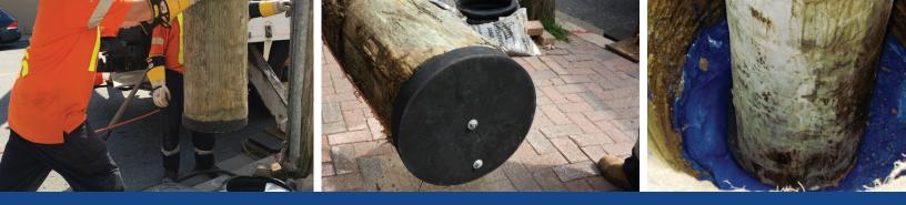
The **ConduDisc**<sup>®</sup> can be used with or without **ConduFlow**<sup>®</sup> pourable backfill. When using **ConduFlow**<sup>®</sup> with the **ConduDisc**<sup>®</sup>, ensure that **ConduFlow**<sup>®</sup> is properly mixed and poured down the hole prior to installing the **ConduDisc**<sup>®</sup>.
