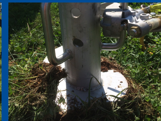
CONNECT GROUND WIRE FROM TRUCK TO SCREW
