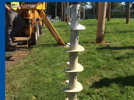
ATTACH SCREW AND INSTALL INTO THE GROUND
