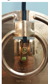
Figure 2: Copper Compression Connector Attachment to the Galvanized Steel Grounding Plate (left and middle) and the ConduDisc Inner Plate (right)
